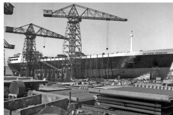
Methane Princess takes shape on the slipway at the Vickers Armstrong yard
