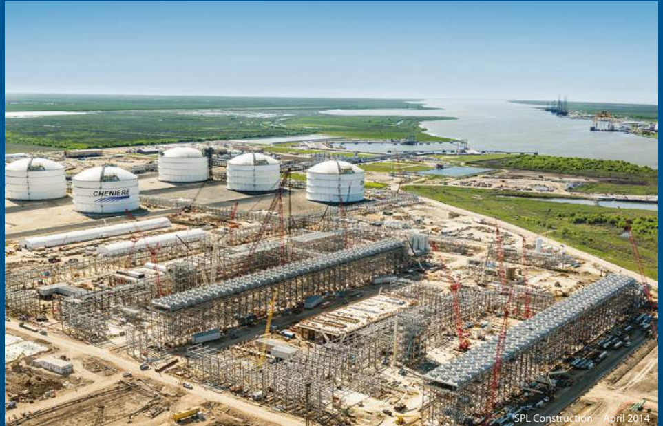
SPL Construction - April 2014
