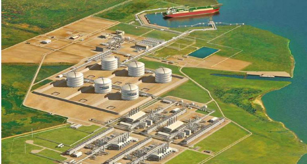
Graphic shows four of the six trains planned for Sabine Pass in place
