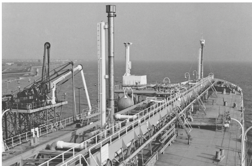
Although built 20 years before the IGC Code was adopted, the Methane ships anticipated the Code's requirements to a startling degree
