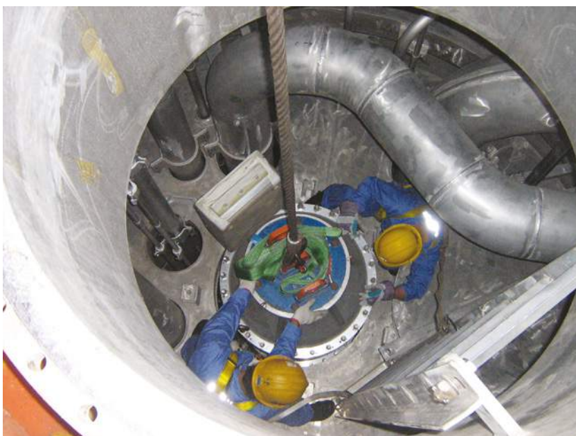
Lifting a cargo pump clear of the tank for servicing
